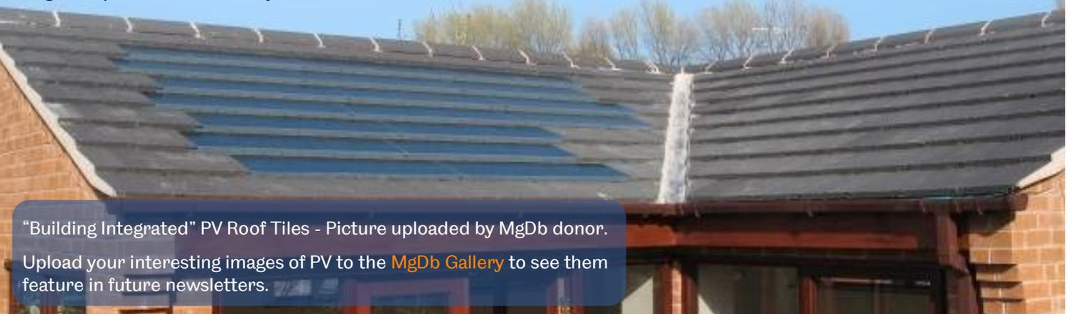
"Building Integrated" PV Roof Tiles - Picture uploaded by MgDb donor.
